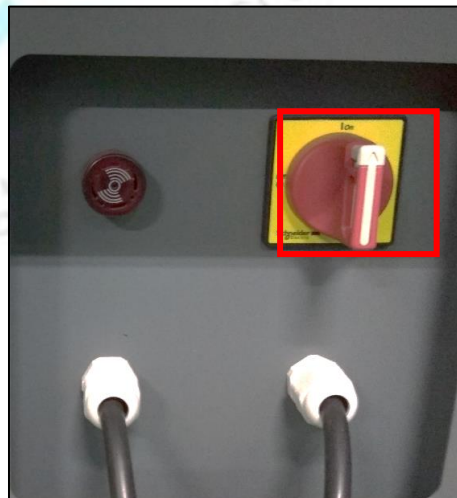
Figure 55: Turn Off the Main Power Button
